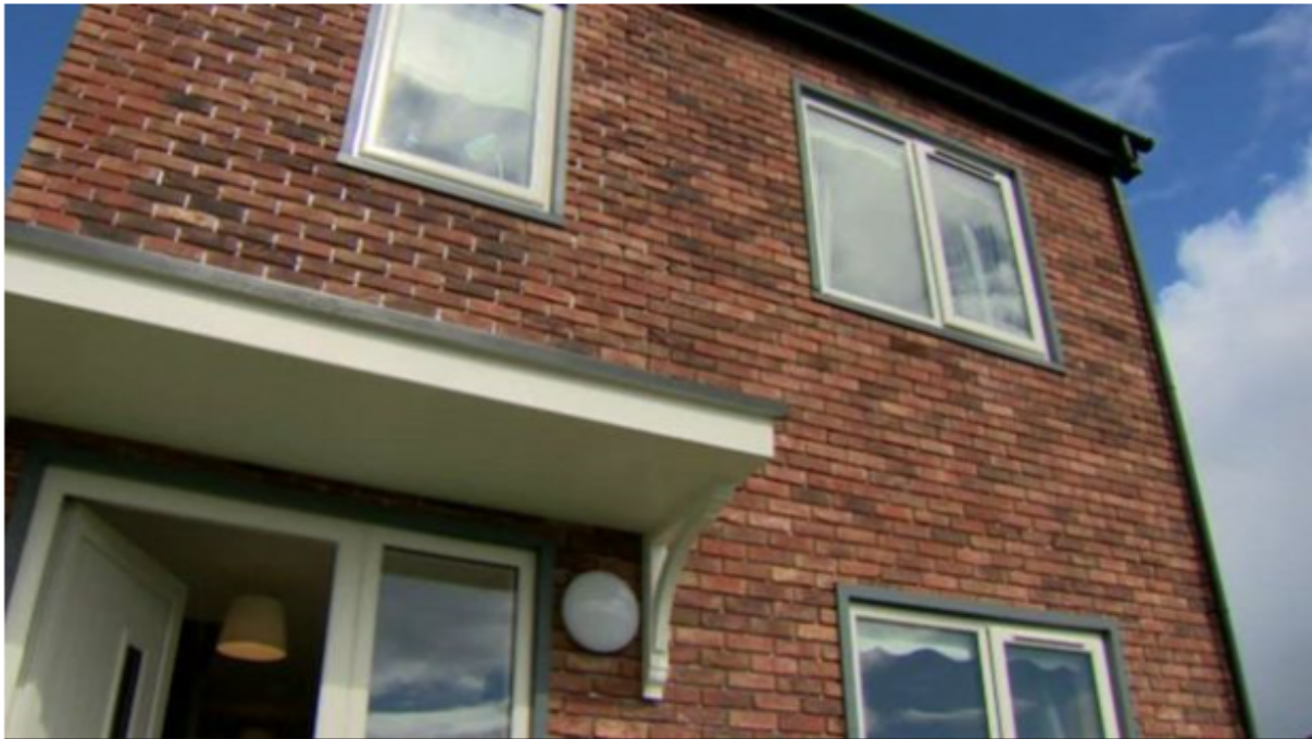
The Clanmil Housing Association says off-site construction could be the future of social housing
