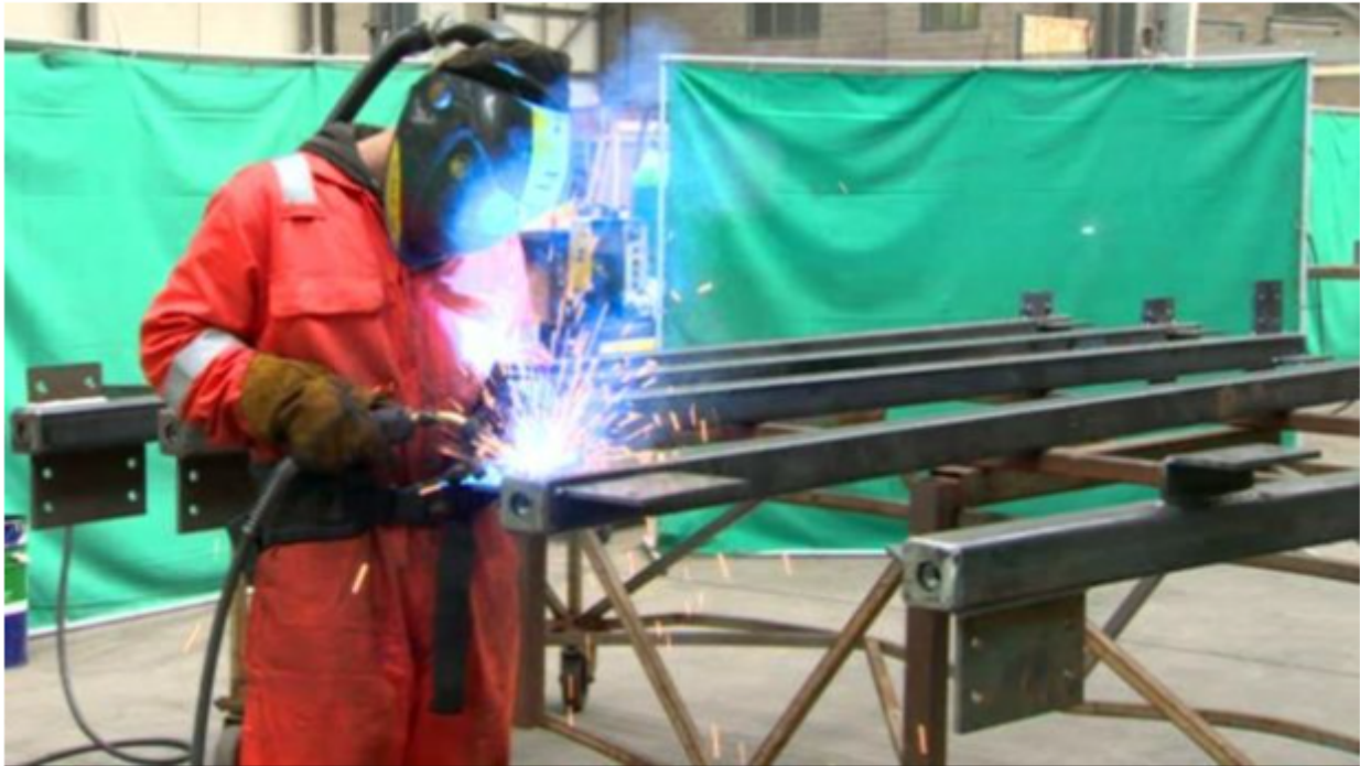
The steel frame buildings are manufactured in a Lisburn factory
